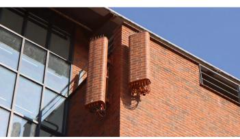
SEKISUI KYDEX offers a suite of thermoplastic solutions to develop a seamless 5G antenna enclosure that houses small cells within one.
